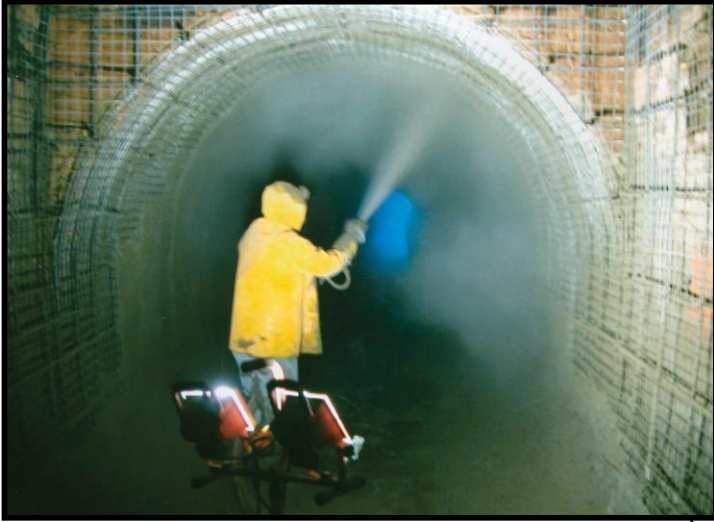
Reinforcement Installed, Ready for Gunite Placement
