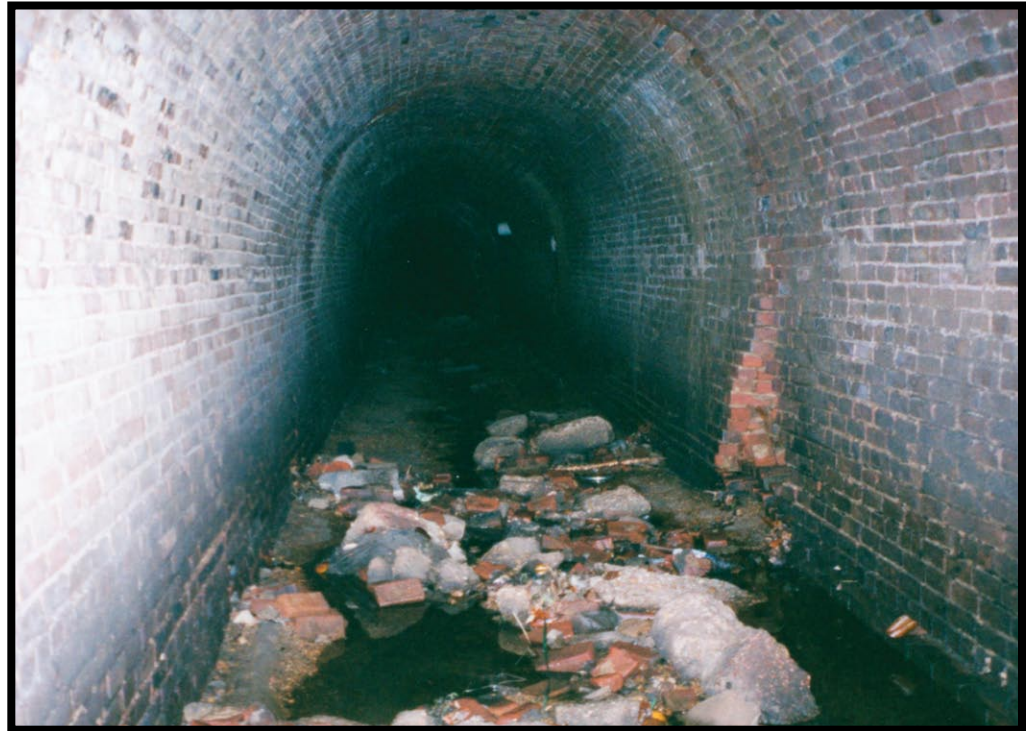
Existing Brick Tunnel
