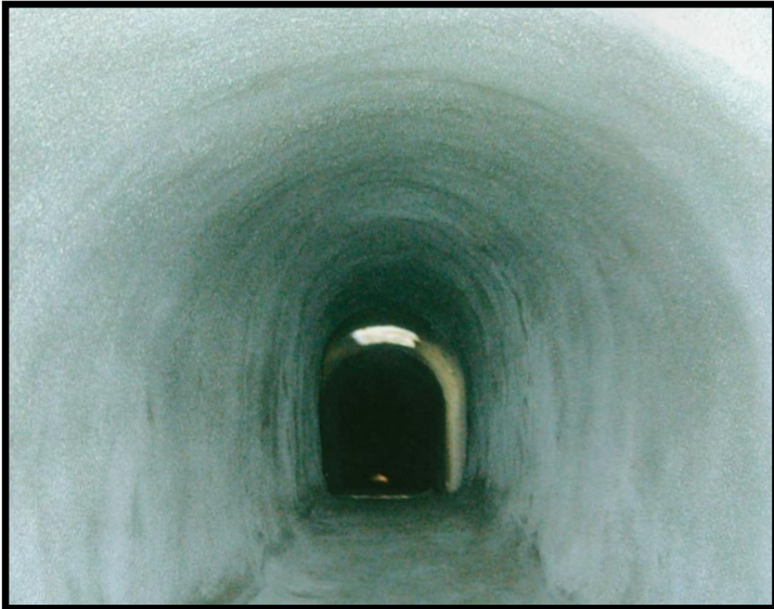
Completed Gunite Lining
